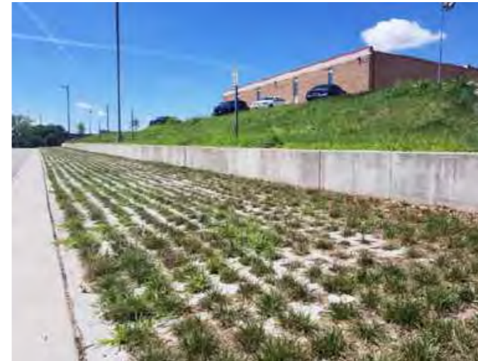
Examples of grasscrete and grass mesh design approaches for temporary grade parking in business/science parks
